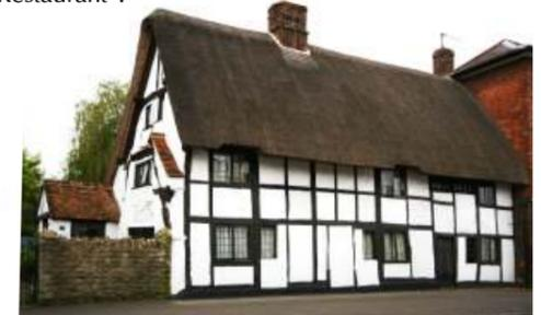
**20** Further along the High Street, **The Cruke** is a beautiful timber framed house of box frame construction and dates from the 15th C. Note the medieval stained glass in the upper right window. The name is misleading as the cruck timbers are a remnant of a previous building.
